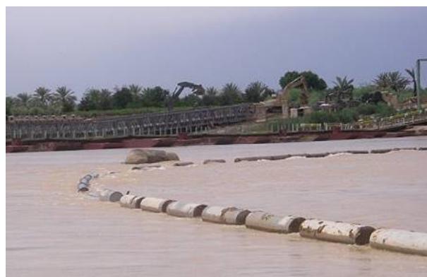
As Sindiyah Bridge and Mine Boom After Repairs
